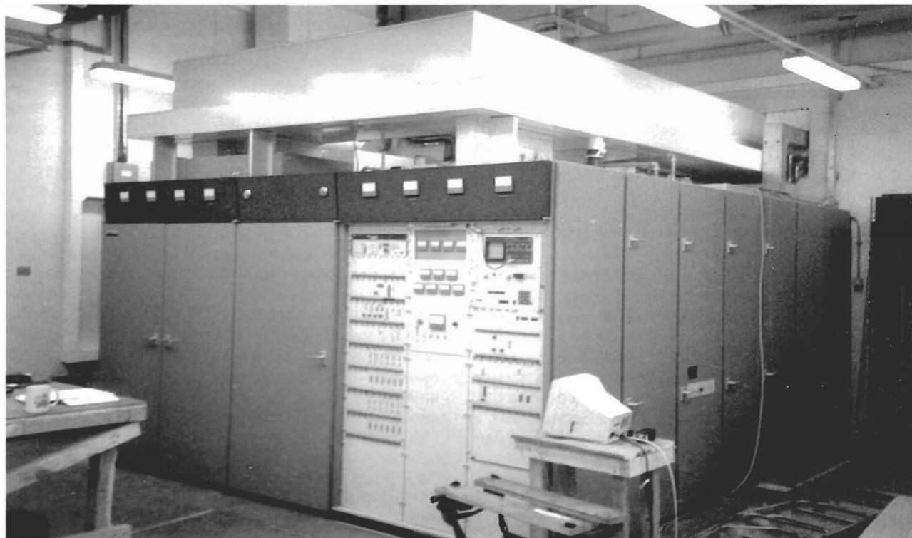
One of the two 250 kW transmitters under test at the East Asia Relay Station.
