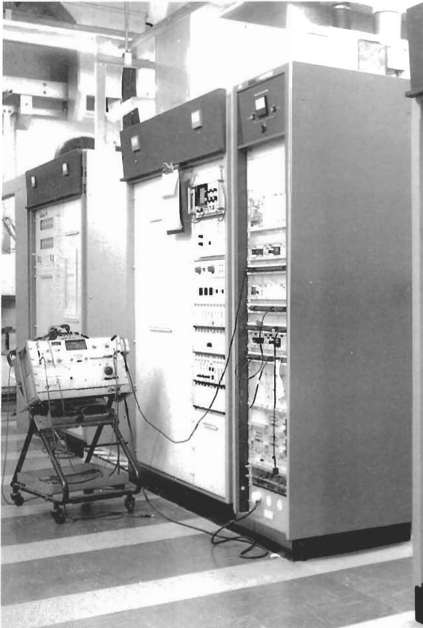
One of the two 250 kW transmitters under test at Droitwich.
